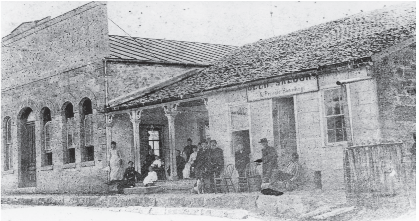
The 1872 photograph clearly shows the building's original porch, a private frontage area that is now used as a public sidewalk and is not ADA compliant.
